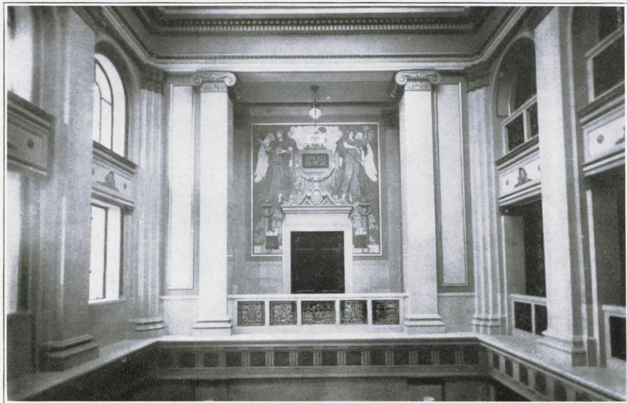
MAIN LOBBY, SECOND FLOOR, WEST—ENTRANCE CIRCUIT COURT
