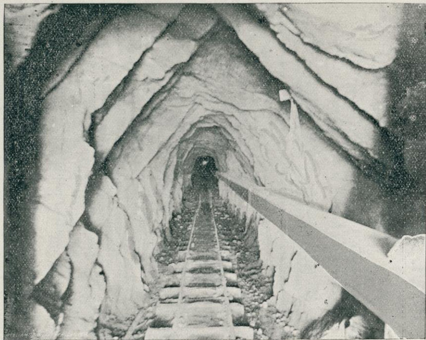
INTERIOR OF A MINING TUNNEL.
