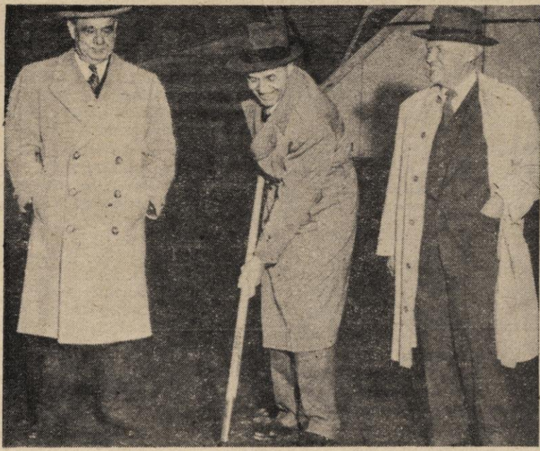
Gov. Walter J. Kohler grins as he chops out the first shovelful of dirt to begin construction of the new intern-resident dormitory for the medical school. Looking on are A. Matt. Werner, left, vice president of the regents, and Dr. Harold M. Coon, superintendent of Wisconsin General hospital. —Photo by Gary Schulz
