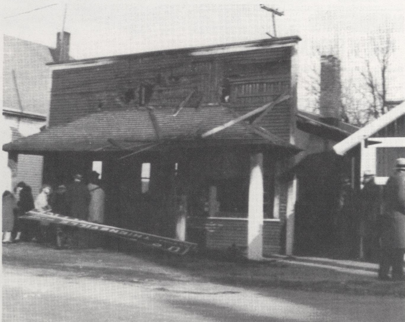
One of the worst fires in the history of the department was the post office fire on New Year's Eve 1933. Postmaster John Albers lost his life in the fire, which destroyed the building.
