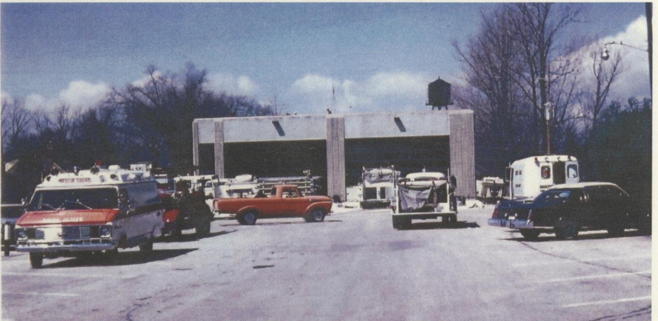
After being housed at the highway department garage for a year, the department moved to the present firehouse, located at 250 Elm Street. This view shows the apparatus floor being readied for the equipment.
