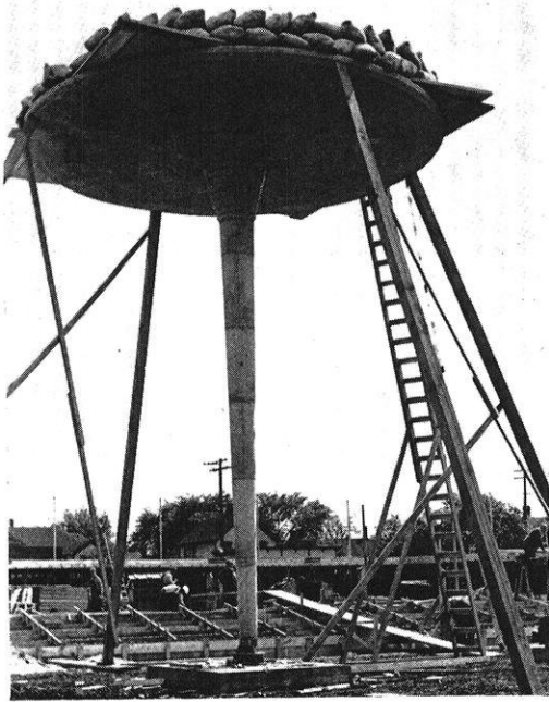
Load Test of Tapered Column
