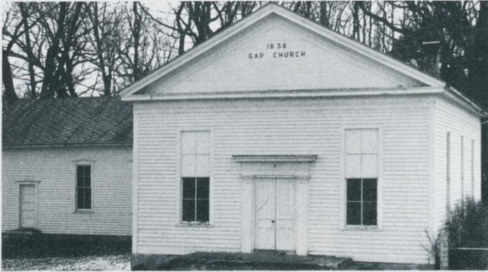
Oldest church in the Albany area is the Gap Church, built in 1858. The church served the community for many years before services were discontinued in 1940.
