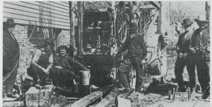
The first community well was drilled next to the old Village Hall in 1914. The well, 368 feet deep, still has a capacity of 475,000 gallons of water per day. Original cost was $16,292.94.
