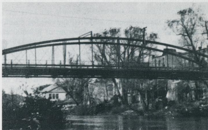
This wagon bridge over Sugar River was a 120-foot long suspension bridge built in 1877 after flood waters had destroyed a series of earlier bridges. In 1923 the bridge was replaced by the present steel reinforced concrete span.
