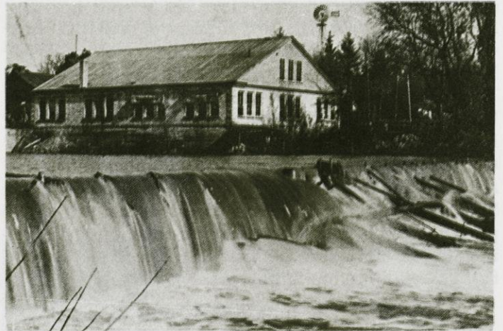
Debris, washed down the river during a high water period, piled up at the base of the dam. Building in background is the latch factory.
