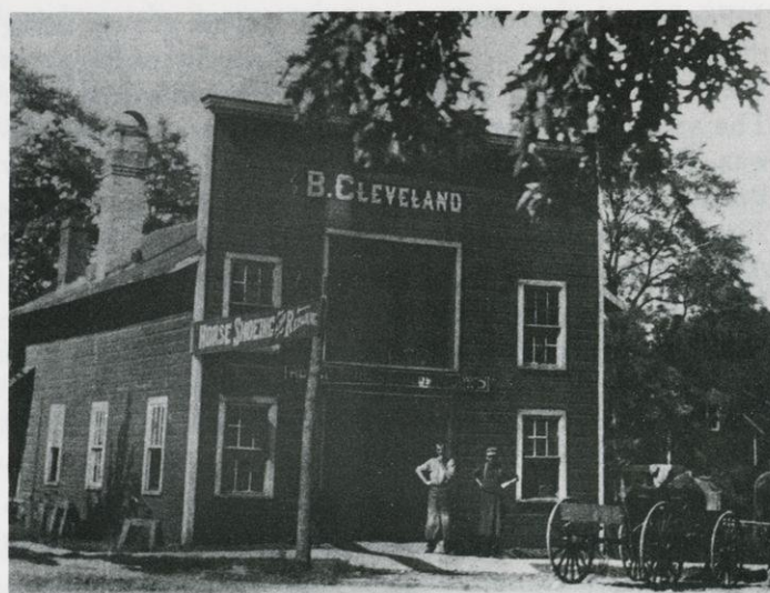
Blacksmith shop operated by Ben Cleveland, Sr., and later by his son, Ben, Jr., still stands on the northeast corner of Main and Mechanic Streets. The building shown here faced south toward Main Street, but was later turned around to face Mechanic Street.
