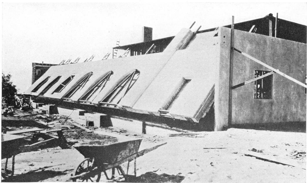
THE WALLS OF THIS CLUB ROOM WERE BUILT HORIZONTALLY, METAL WINDOWS AND DOOR FRAMES PUT IN POSITION AND THE WHOLE TIPPED INTO PLACE AND FASTENED SECURELY AT THE CORNERS: SUCH CONSTRUCTION MATERIALLY REDUCES THE COST OF THE BUILDING, WHILE MAKING IT ALMOST IMPERVIOUS TO TIME AND WEATHER.
