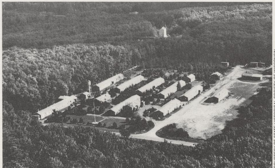
Civilian Conservation Corps camp at Devil's Lake State Park. Conservation base operations were headquartered at eight camps in state parks and 40 other locations in Wisconsin.
