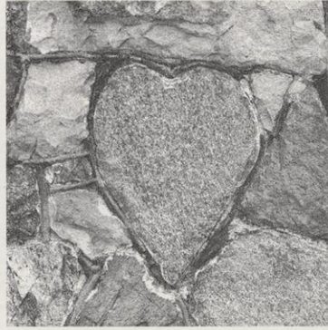
masonry at Poynette Game Farm
