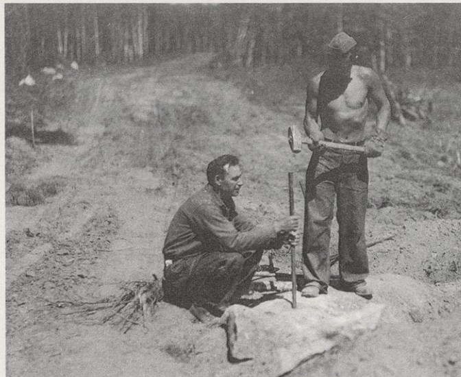
Paving the way for CCC. Chiseling the charge holes to blast the road leading to the White Sand CCC Camp, Crystal Lake, Vilas County, May 1934.
