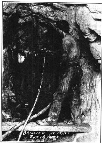
Preparing a Blast in a Mine at Butte, Montana.
