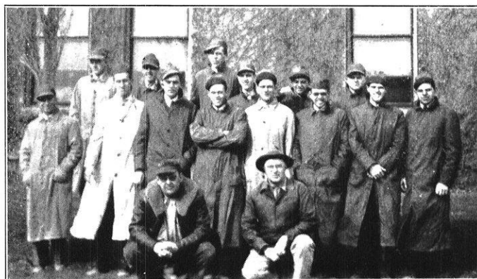
Bring on your Cement Plant.
