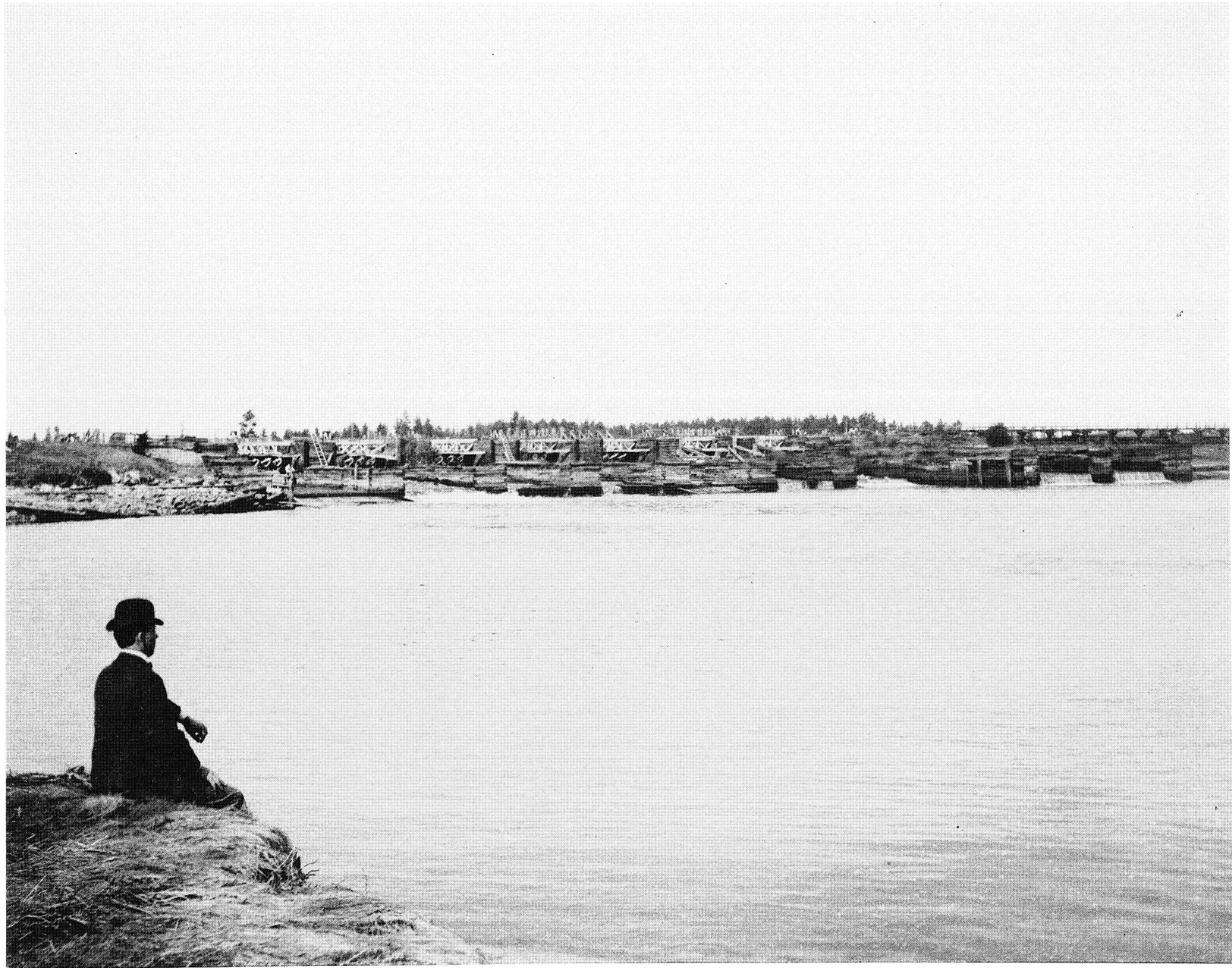
WISCONSIN RIVER DAM—TOMAHAWK.
