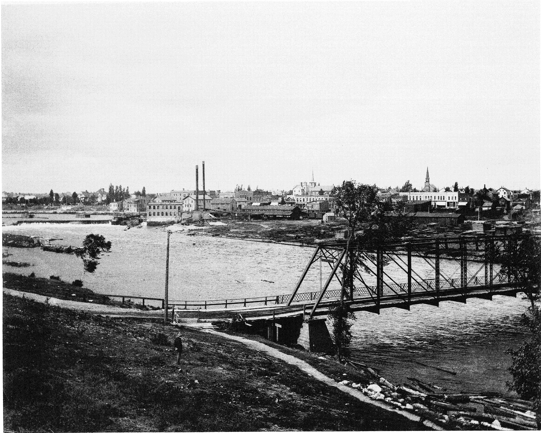
VIEW OF MERRILL—EAST SIDE.
