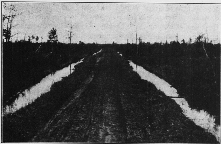
Fig. 8. DIFFICULT ROAD MAINTENANCE
