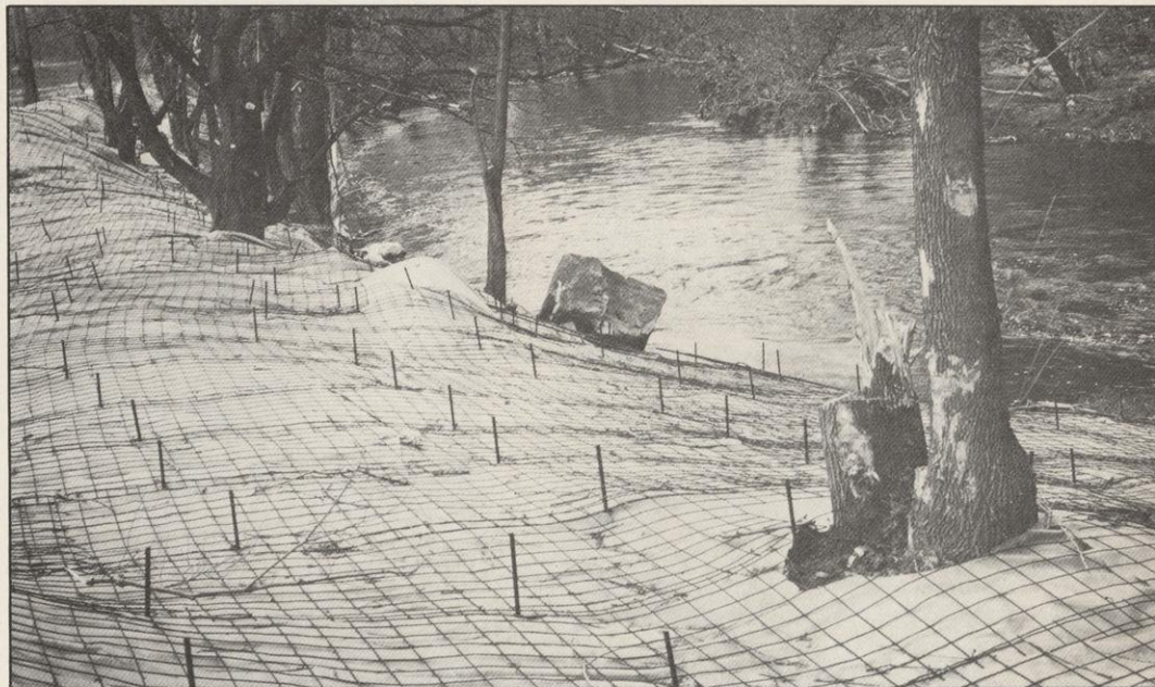
The shoreline of the Sheboygan River was covered with a special mesh last winter to prevent erosion of PCB-contaminated soil. Tecumseh Products Company has removed 106,000 cubic feet of soil under DNR order to make the site safe again. The firm had dumped sweepings from its engine manufacturing process along 500 feet of shore.
