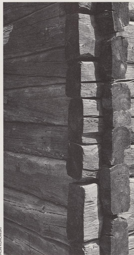
Grooved notching kept Scandinavian-designed cottages sturdy and tight.
