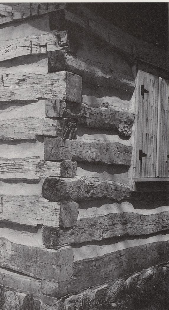
Each culture brought distinct construction techniques. The chinking, corner design and log arrangement in the Gotten cabin typify German building methods.
