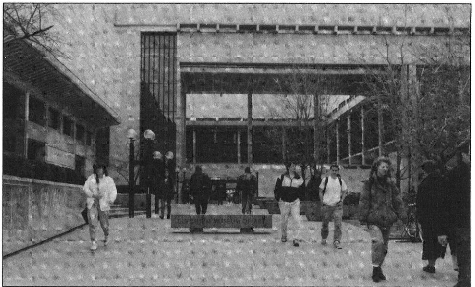
The inner mall of the Humanities Building.
