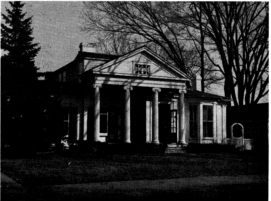
FIGURE 7. 1247 South Main Street (photograph by Todd Dahlen and Peter Vallone).
