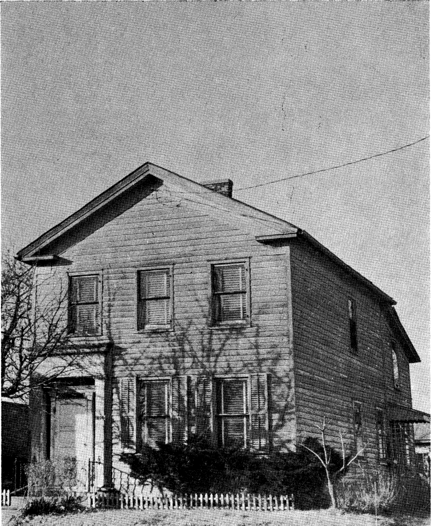
FIGURE 3. 1108 Douglas Avenue before recent renovation (photograph by Todd Dahlen and Peter Vallone).
