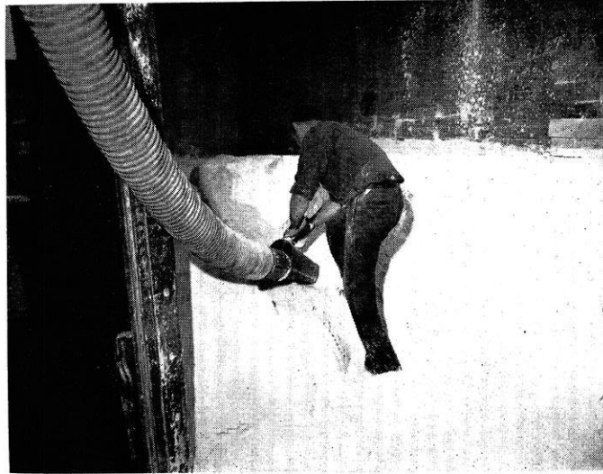
Pneumatic Hose —Engineering knowledge is important to the work of the hygiene staff. This apparatus is used to suck up powdered ceramic materials from freight cars to large storage silos. The workman is thus protected from dust which would be unavoidable if the powdered material had to be shoveled.
