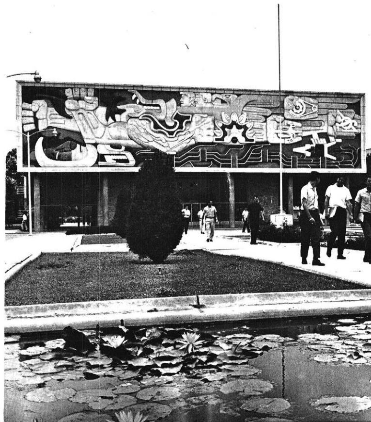
Administration Building on the Monterrey Tec Campus.
