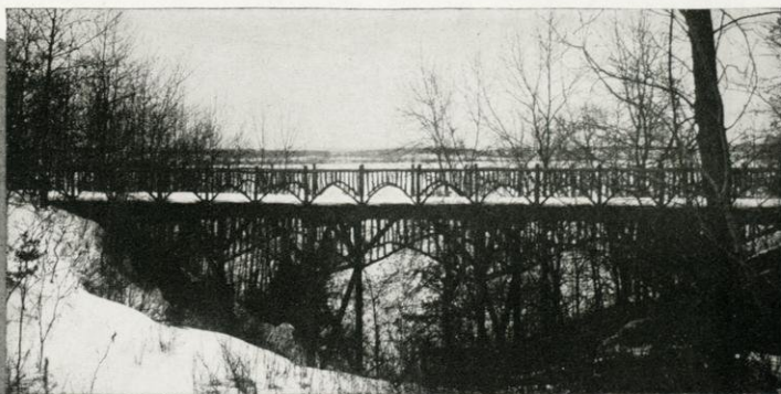
Rustic Bridge, Lake Mendota Drive
