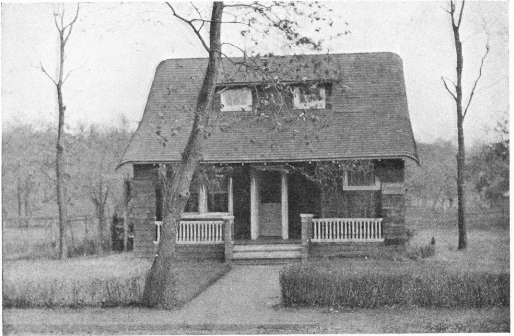
THE ROOF LINE OF THIS BUNGALOW IS MADE IN IMITATION OF THATCHED ROOFED ENGLISH COTTAGES.
