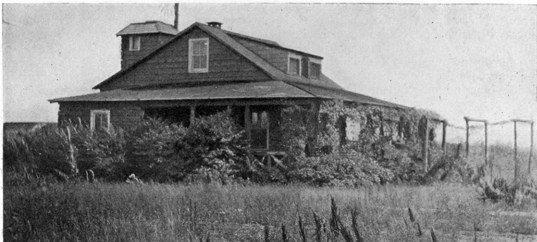
A BUNGALOW ENCLOSED WITH BOARDS WHICH ARE ALLOWED TO PROJECT LOG-CABIN FASHION AT THE CORNERS.
