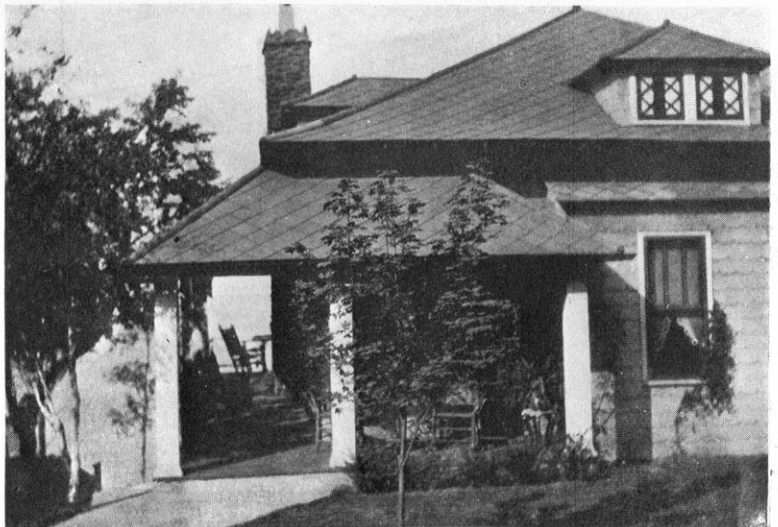
BUNGALOW BUILT TO GIVE VIEW OF THE RARITAN BAY FROM THE PORCH.
