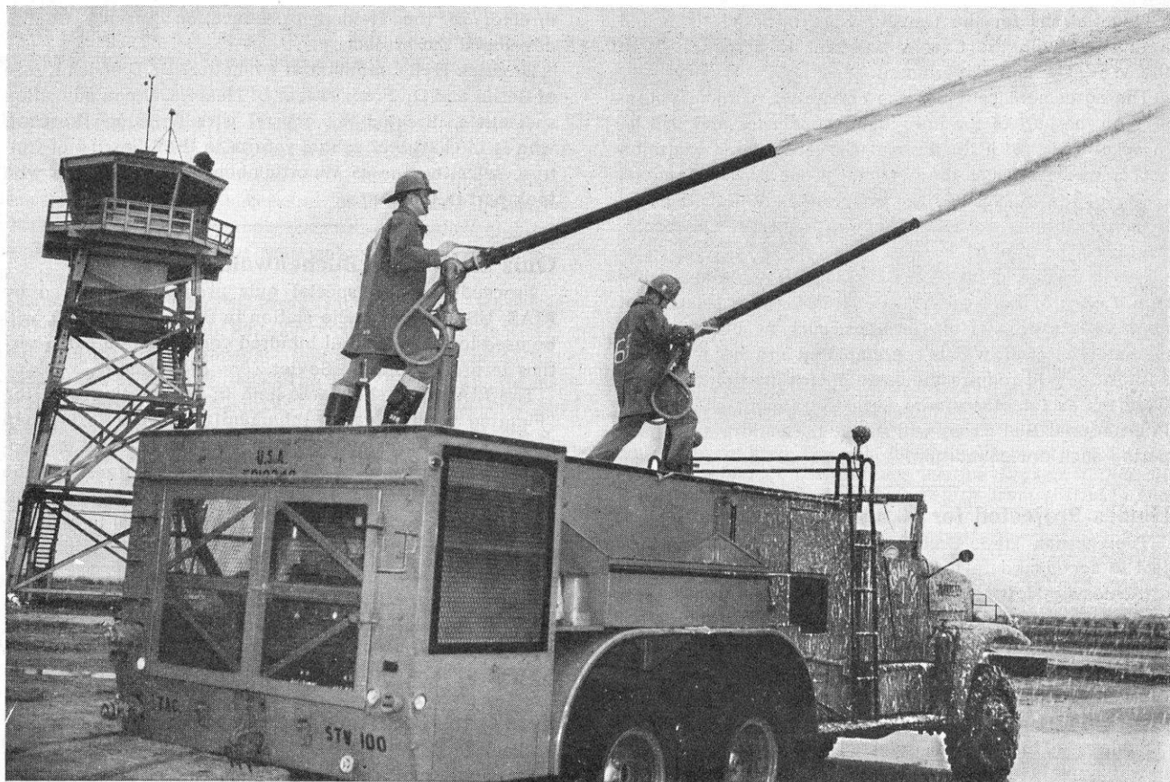
A fireman can't afford to go wrong so Rhine/Main firemen do daily drills with their foam guns to be sure they spray properly. The foam — protein base liquid — prevents oxygen reaching the blaze thus extinguishing the flames. (USAF photos)
