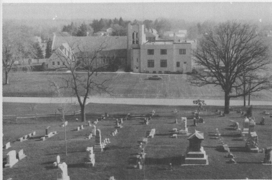
Norway Ev. Lutheran Church as viewed from Indian Hill
