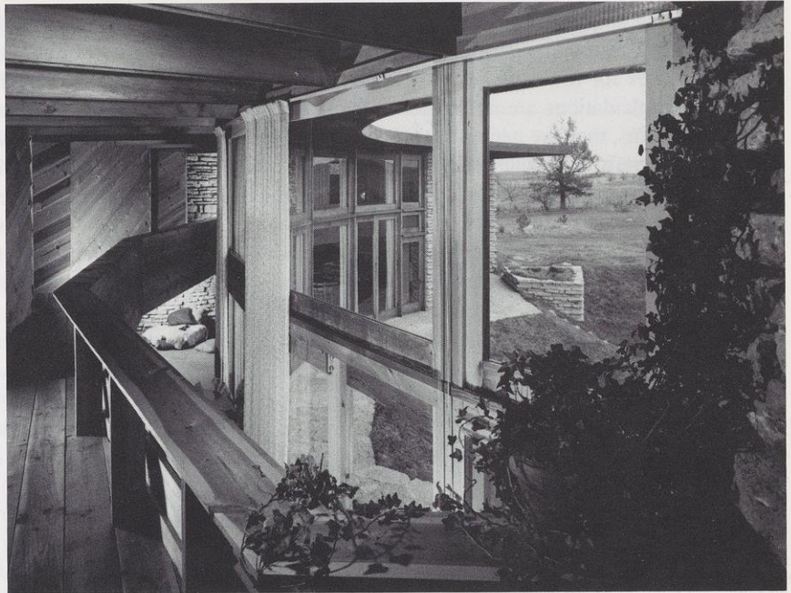
The mezzanine bedroom level. The balcony is suspended from the roof joists, leaving the main floor clear of structural support members. The December winter sun reaches the top of the balcony railing. Copyright Ezra Stoller, ESTO. Used by permission.
