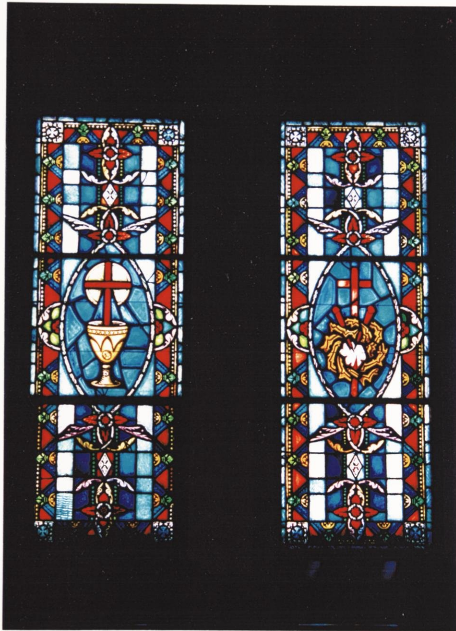
Window 2, north wall
