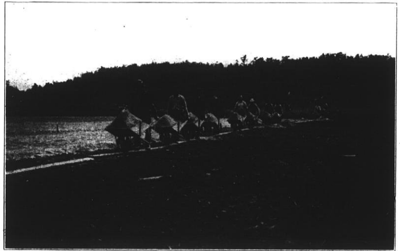
Bog construction on the Chas. L. Lewis bog at Shell Lake, Wis.
