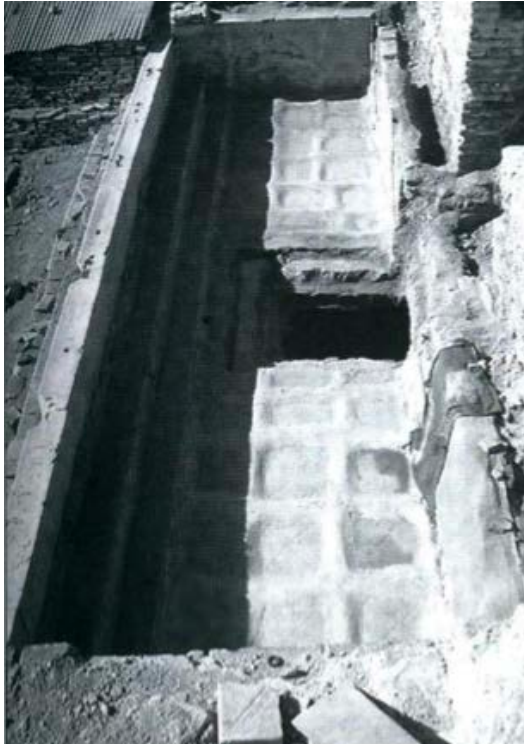
Figure 4.43: Interior view of the pool in the eastern bay of Caldarium III with the negative imprint of the testudo alvei.
