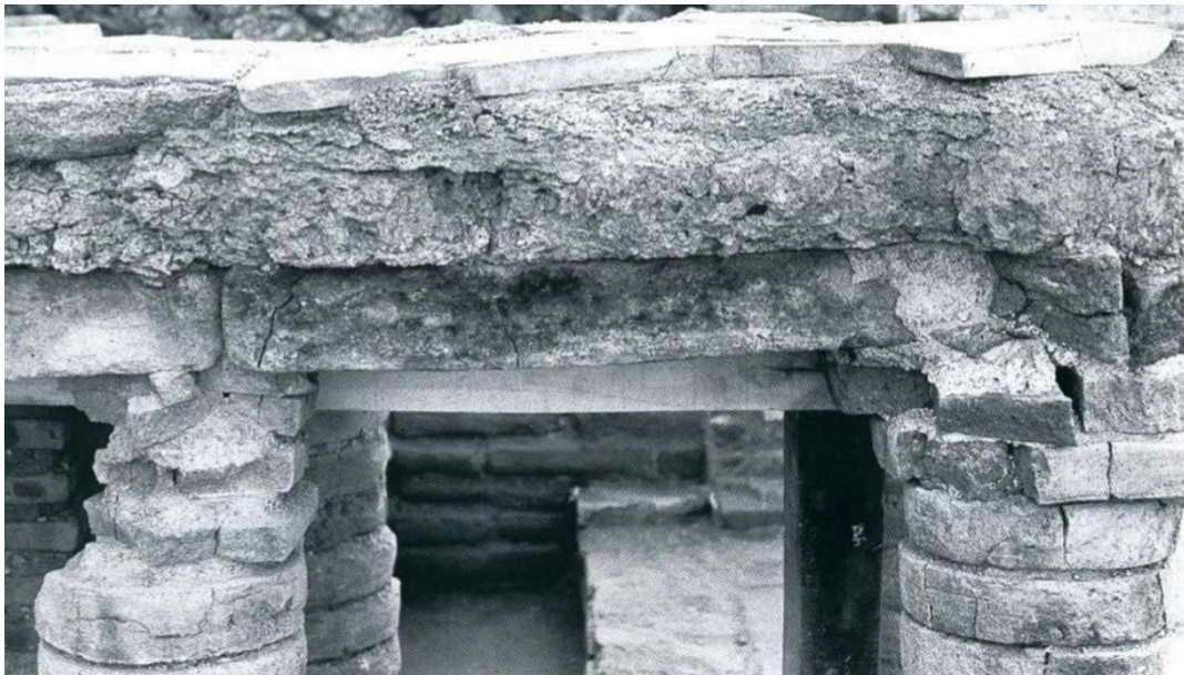
Figure 4.14: View of the double mortar layer between the caldarium floor and the supporting pillars [in Caldarium I].
