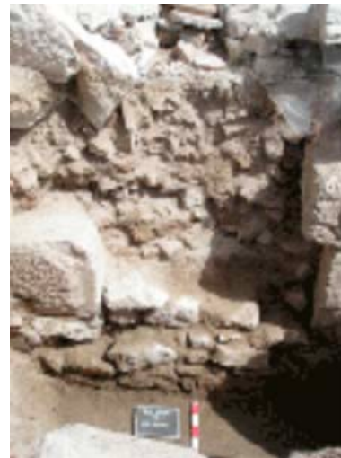
Figure 4.53: View of the crack in the foundations with sixth century A.D. repairs.
