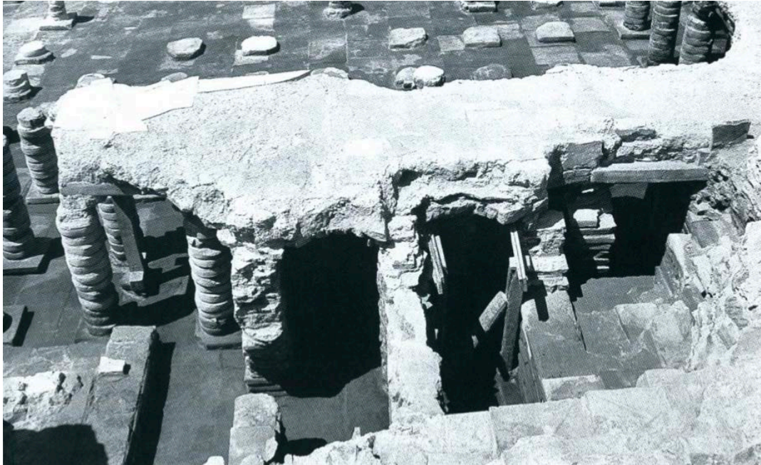
Figure 4.13: Preserved hypocaust pillars in the southeast corner of Caldarium I.
