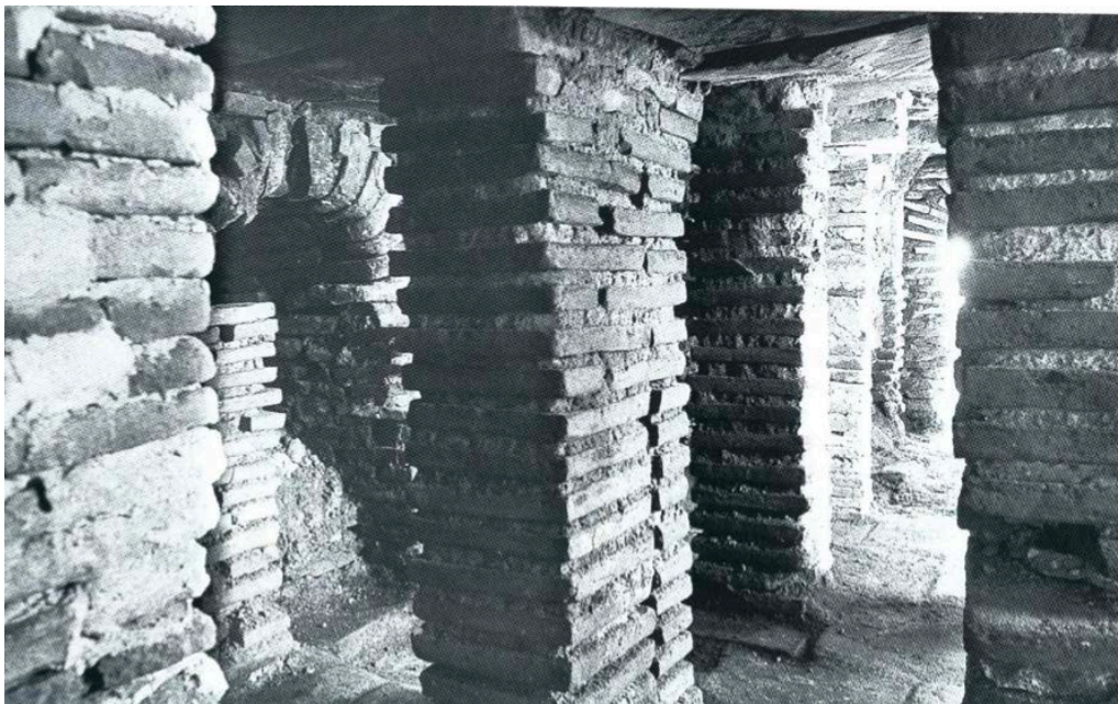
Figure 4.46: View inside the hypocaust system below Caldarium III.
