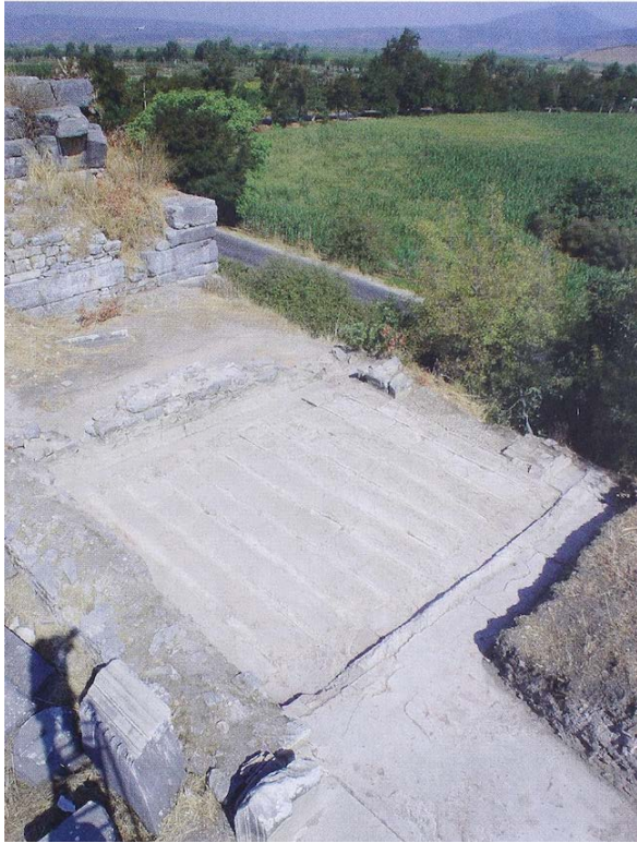
Figure: 3.61: Roof consisting of terracotta tiles and opus signinum constructed on the floor of burnt-out Room XXII to protect the basement rooms – mostly Room E – from water penetration.
