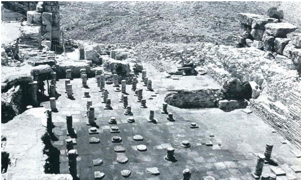
Figure 4.10: View of Caldarium I from the north with exposed hypocaust pillars under the floor. Notice that most of the hypocaust pillars are round, but there are some square ones towards the back. The square hypocaust pillars are thought to be contemporaneous with the transformation of the Marble Hall to Caldarium III, when square hypocaust pillars were also installed underneath the floor in C III.
