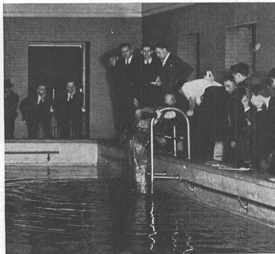
Cutting iron under water Showing young engineers how it's done
