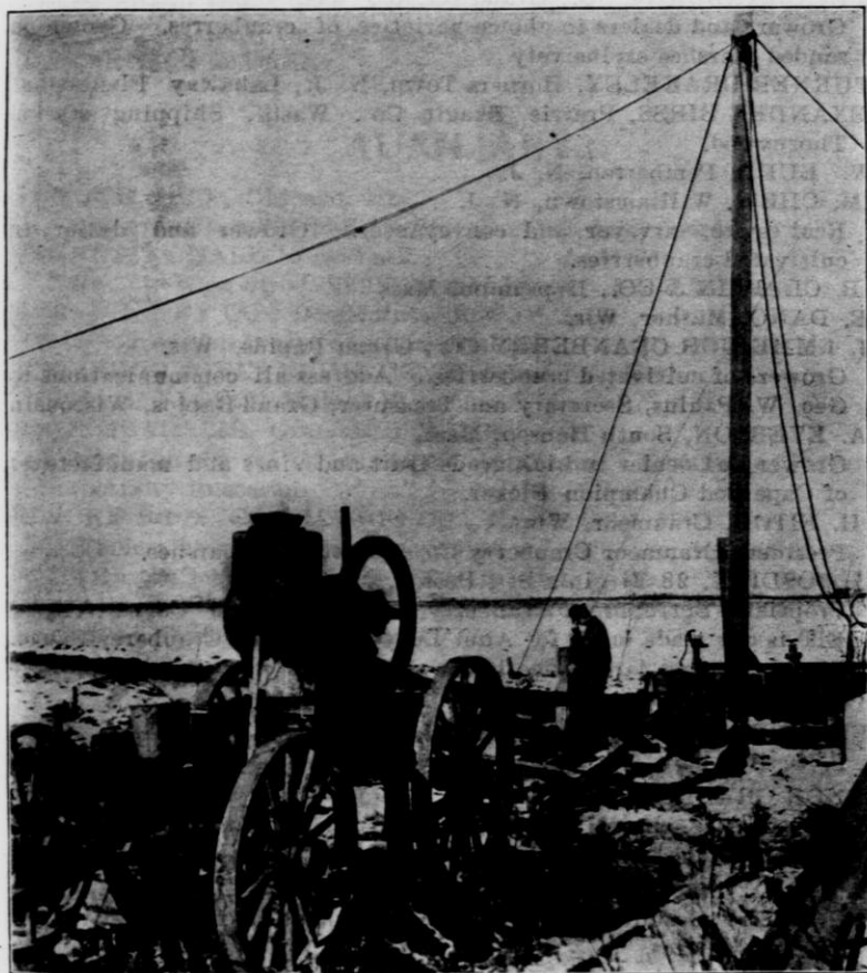
Six H. P. engine left on wagon during test—Notice one pole, three rope derrick ("Jim pole") 26 ft. high.
