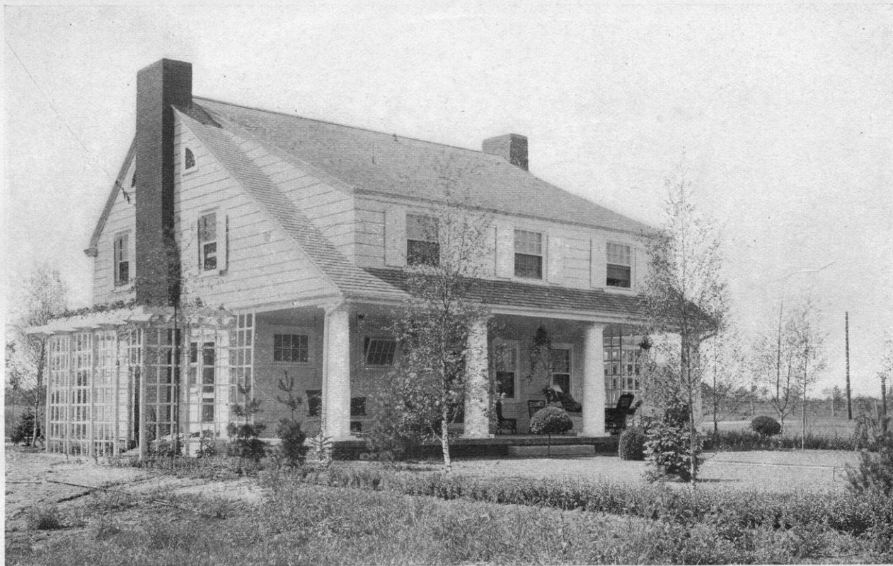
VIEW OF THE REAR OF THE HOUSE, SHOWING PORCH, MOST INTERESTING ROOF CONSTRUCTION AND LAT- TICED PORCHES AT EITHER END OF THE DWELLING.
