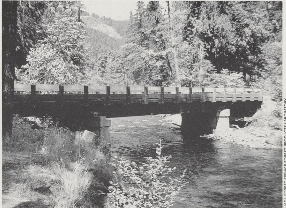
Wood bridges blend gracefully into rural landscapes. Modern construction methods, strength and low cost make wood bridges a good choice for spans up to 60 feet long.
