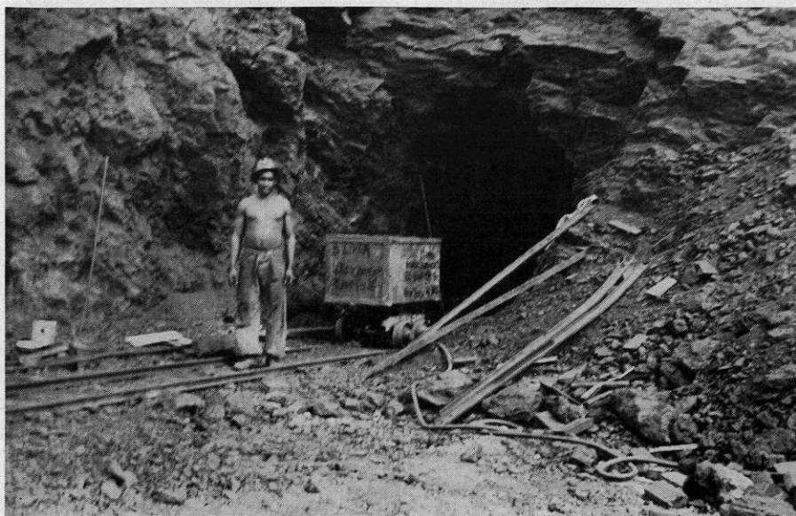
A VIEW of the mouth of the exploration tunnel on Cerro Bolivar. This investigation of the mountain led U. S. Steel officials to estimate that the ore deposit is worth $10,000,000,000. The tunnel is driven through solid, high-grade iron ore.
