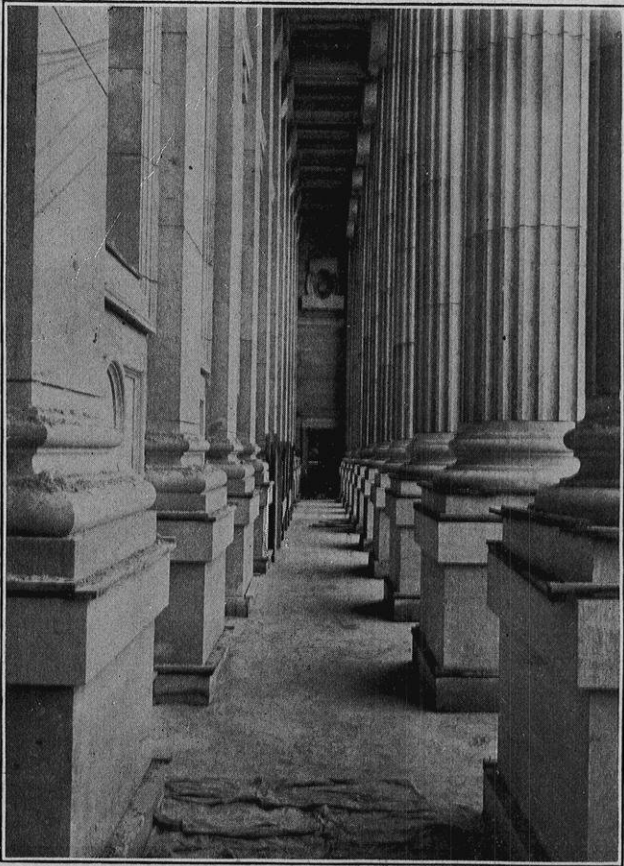
View of East Loggia.
