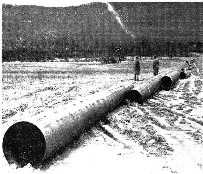
Pipe sections are strung along the right-of-way by heavy trailer-trucks. —Photograph courtesy A. O. Smith Co.
