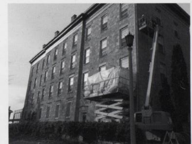
North and South Hall stonework restoration
