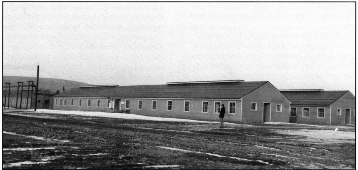
Badger Village Barracks apartment building, 1947
