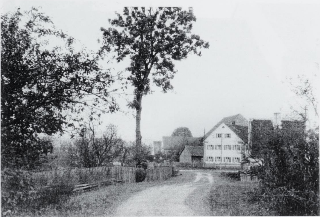
Road leaving the Krause house and barn towards the main road.
