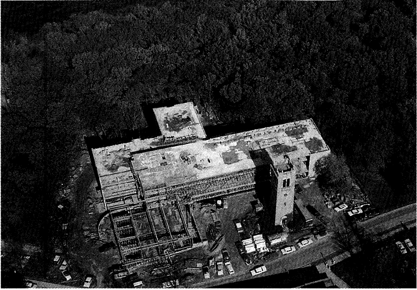
Social Science Building under construction, October 27, 1961. UA, 5292-M.
