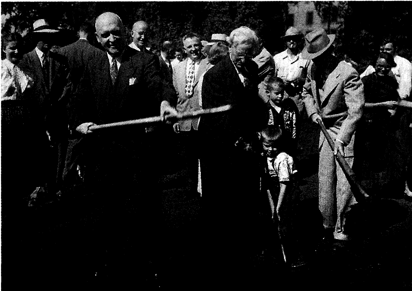
Memorial Library ground-breaking ceremony, July 24, 1950; l-r: E.B. Fred, Regent Daniel H. Grady, Frederick V. Platz, Jr., Regent W.J. Campbell (foreground), O.T. Havey (electrical contractor, smiling in glasses). UA, 1824-M.
