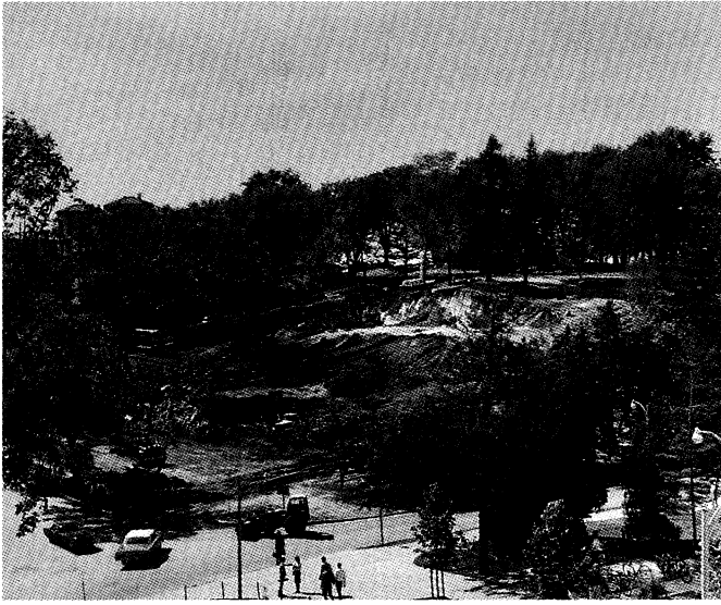
Excavating for Van Hise Hall. UA, X25-3374.
