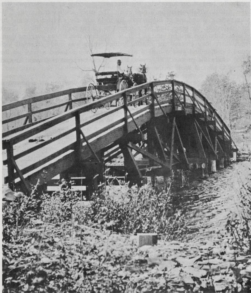
Bridge built by Stout at north end of Hemlock lake, built high to allow boats to pass under it.
