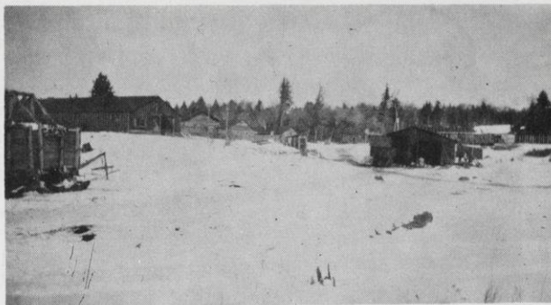
The camp at Winter. At left is the tank for icing the roads. The large building is the cook shanty. Right foreground is the steam hauler shed.
