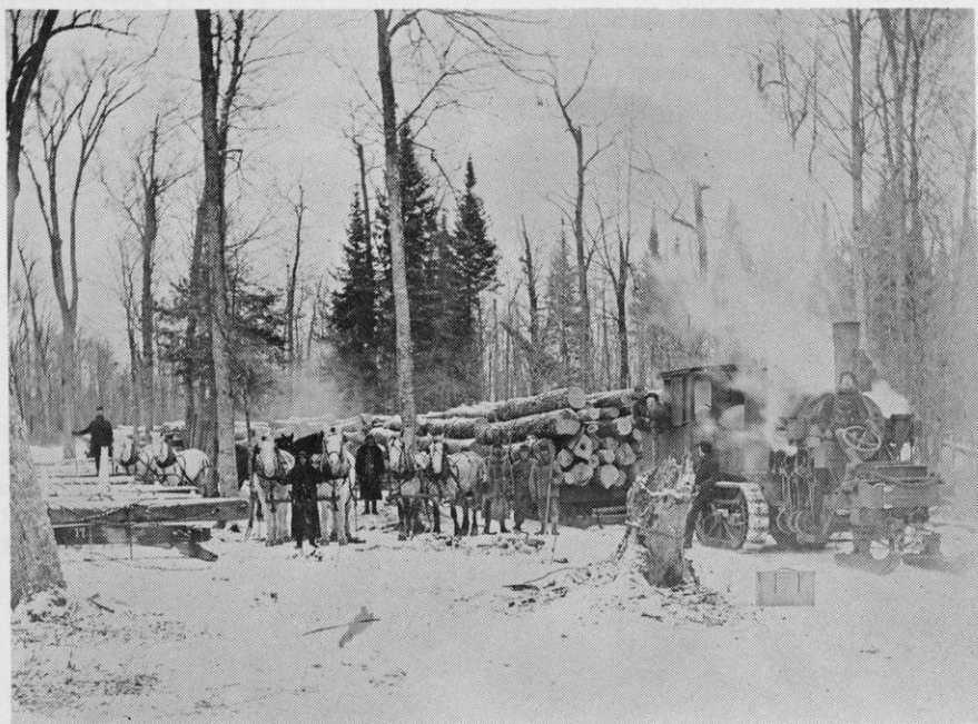
Arpin's steam hauler, Ed Skar driver. Notice the wide sleds at left.
