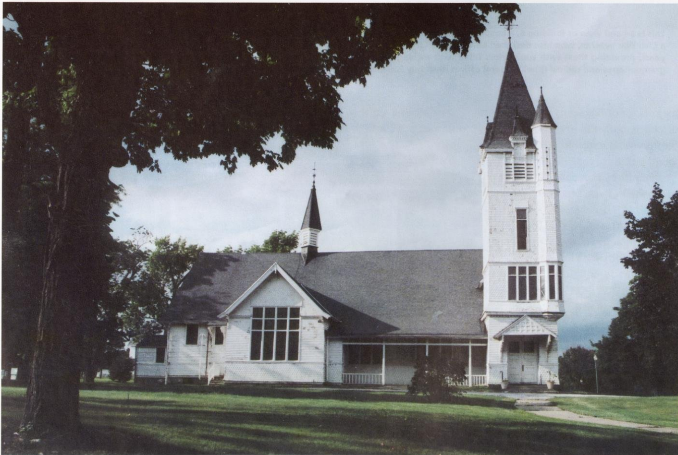
The multi-denominational chapel (1889) was built by soldiers who wanted a separate church structure and who contributed their own resources for its construction. Both Protestant and Catholic services were held there. It is in dire need of restoration.
