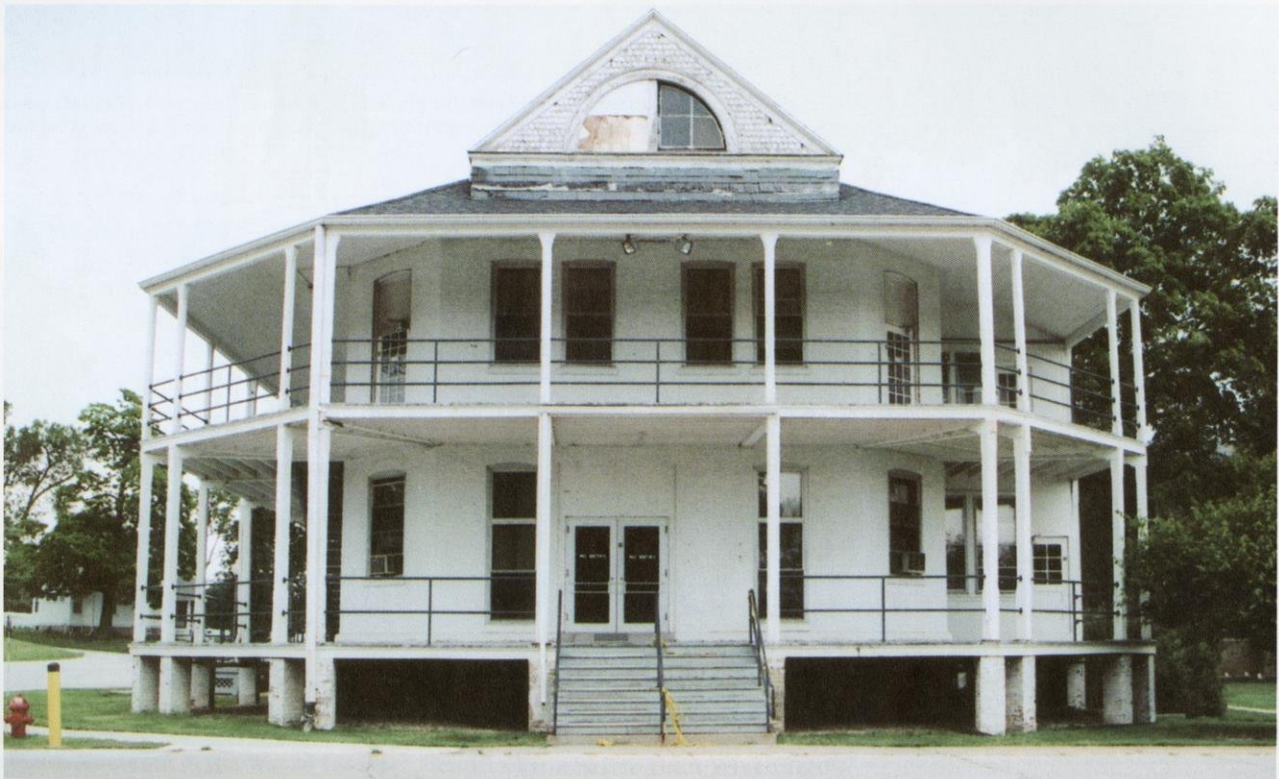
This is an end view of Building 6, a hospital and convalescent ward, built in 1879 and designed by Milwaukee architect Henry Koch, himself a Civil War veteran, who also designed Milwaukee's City Hall and Turner Hall. The third hospital on the grounds, it held elderly veterans for years, providing them with sun parlors filled with rocking chairs, easy chairs, writing desks, flower stands, canaries, goldfish, and early gramophones and radios. It held federal offices until July 2004, when it was vacated.
