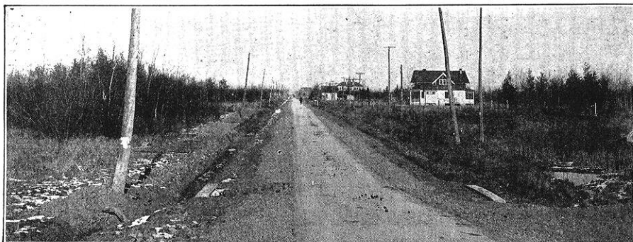
Tower Avenue Road, Superior, Wis. Length 10,500 feet—Width 9 feet. One course 8 inches thick at crown, 6 inches at sides. CHICAGO-AA used.
