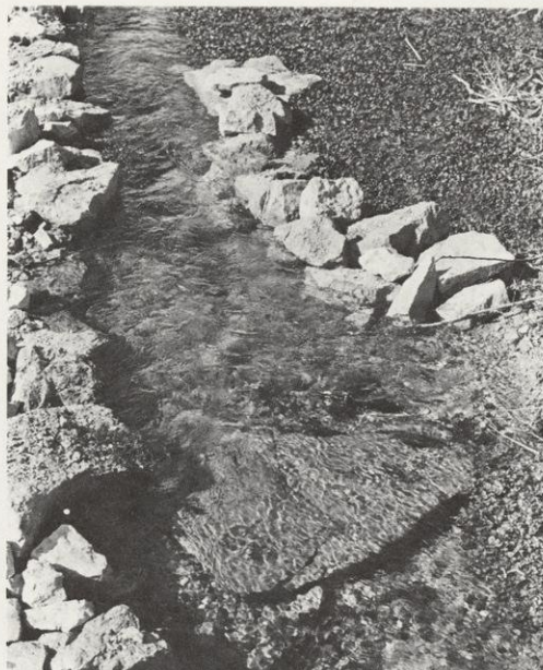
Riprap installed along Bohn Creek, a Trout Unlimited stream project in Iowa County.
