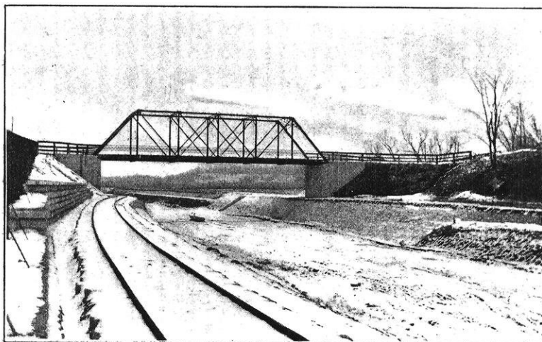
Illustrations of Concrete Construction.
