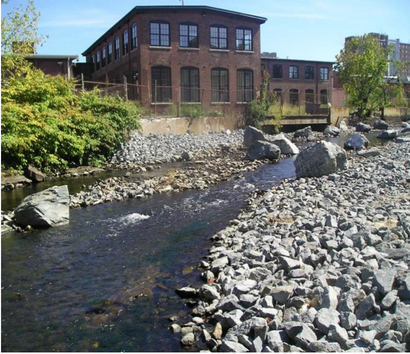
Figure 18: Paragon Dam dam removal after looking west & upstream (above).
