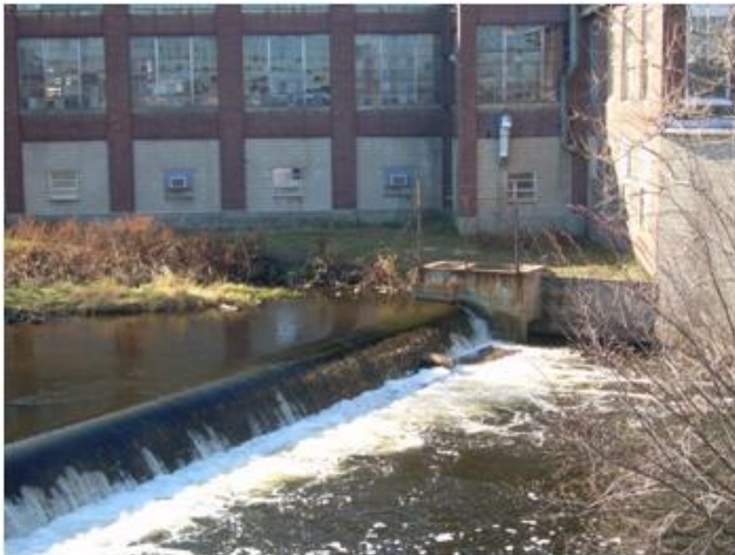
Figure 17: Paragon Dam prior to removal, looking west (above).
