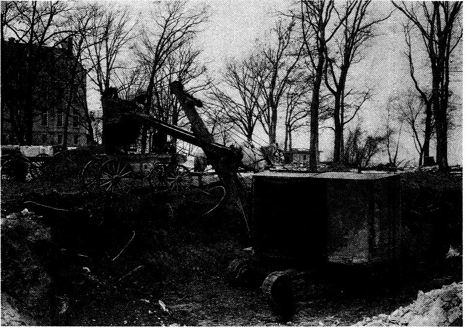
Starting construction of the Memorial Union December 9, 1925
