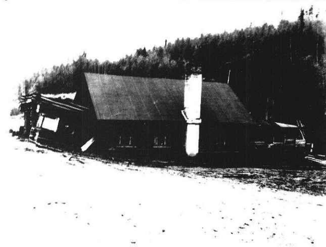
Geological Survey Building, south of Fairbanks, Alaska on Richardson Highway, subsiding because of thawing permafrost.
