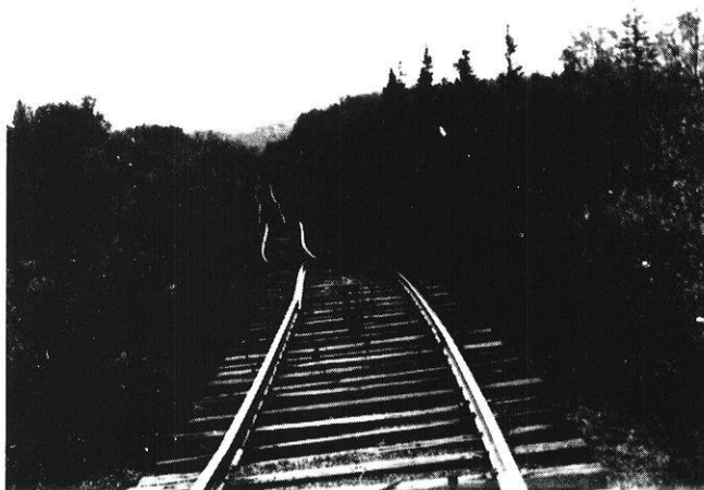
"Roller-Coaster" railroad near Strelne, Alaska caused by differential subsidence stemming from thawing permafrost.
