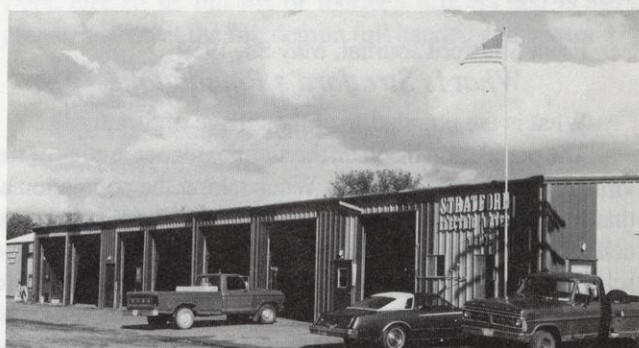
Current Electric and Water Department and Village Garage.
