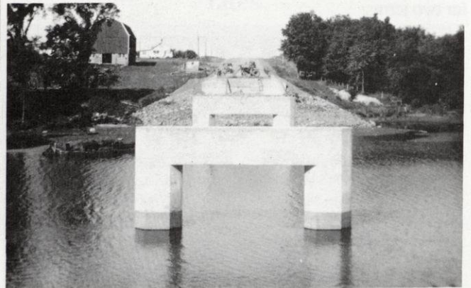
Building the new Bradley Bridge, 1950's. Courtesy Clarence Kafka
