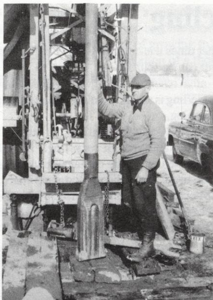
Pete Weber drilling Village test wells. Courtesy of Don Weber.
