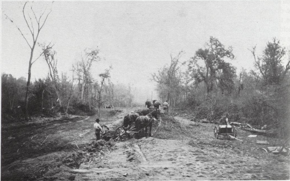
Wheel scraper clearing the Marathon County Railroad bed. Courtesy of The Connor Family
