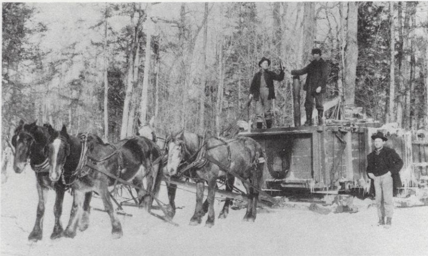
A water tank sleigh. Ice roads were needed to keep loaded lumber sleighs moving. (L-R) Otto Schultz, Otto Sievert and Mike Baltus. (Note stove to keep water from freezing) Photo provided by Connor family.
