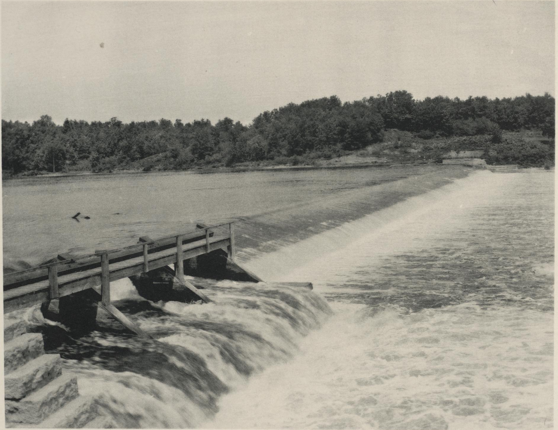
DAM NEAR WRIGHTSTOWN.
