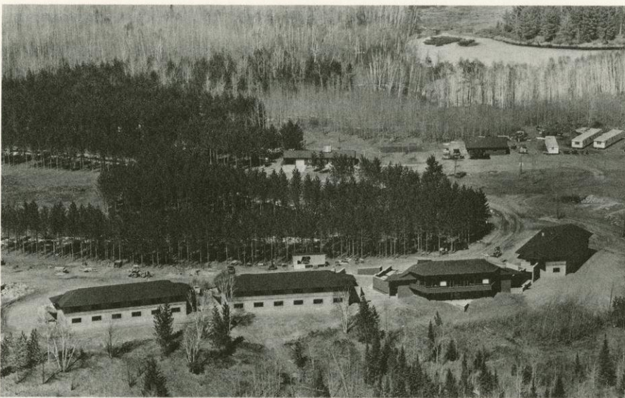
Treehaven field station near Tomahawk while under construction.
