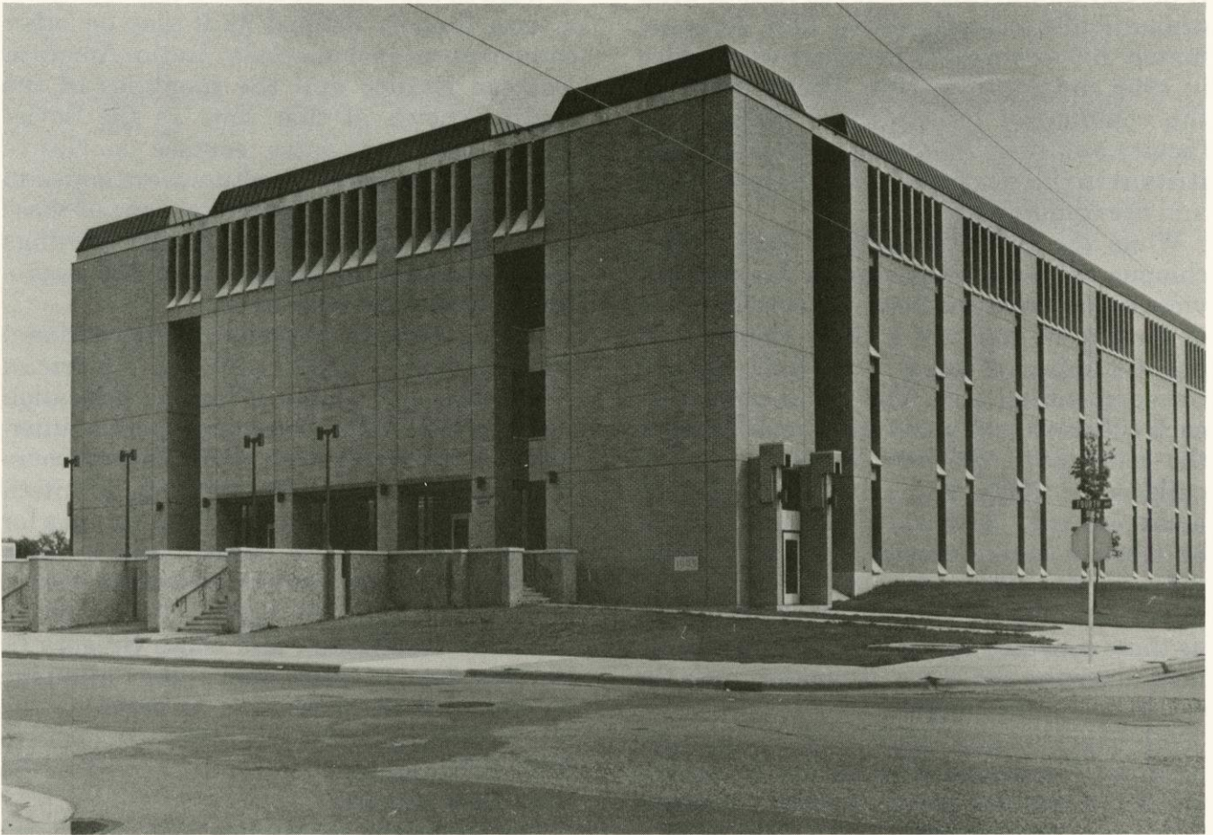
Collins Classroom Center
