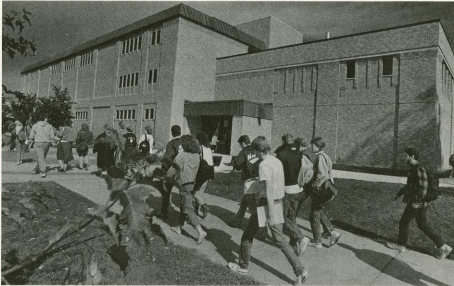
Paper science wing on the southwest corner of the Science Building.
