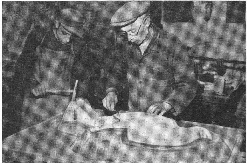
Workmen in a Frankfurt foundry prepare a mold for the casting of the Dove of Peace, which will be erected at the Rhine-Main Airport. The symbolic figure was made by Grete Fendel, Frankfurt sculptress. In its final form it will be ringed by two airplane models. (DENA-Bild)
