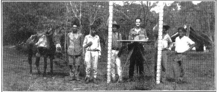
The plane table crew at a camp near the Rio Palmar. Note the metric stadia rods.
