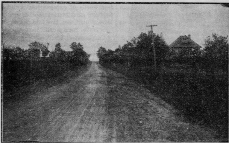
Macadam road in Dane Co. near Madison. Cost (contract), 52 cents per linear foot nine feet wide. Planned by Highway Division, Wisconsin Geological Survey.
