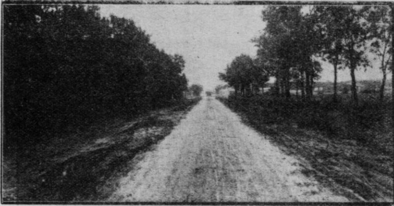
Granite road bound with limestone screenings, near Almond, Portage County. Nine foot stone surface on sand. Experimental road built under the supervision of the Highway Division, Wisconsin Geological Survey.
